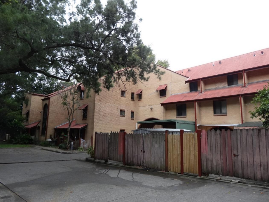
Figure 5: The rear of the site viewed from the existing hardstand area
