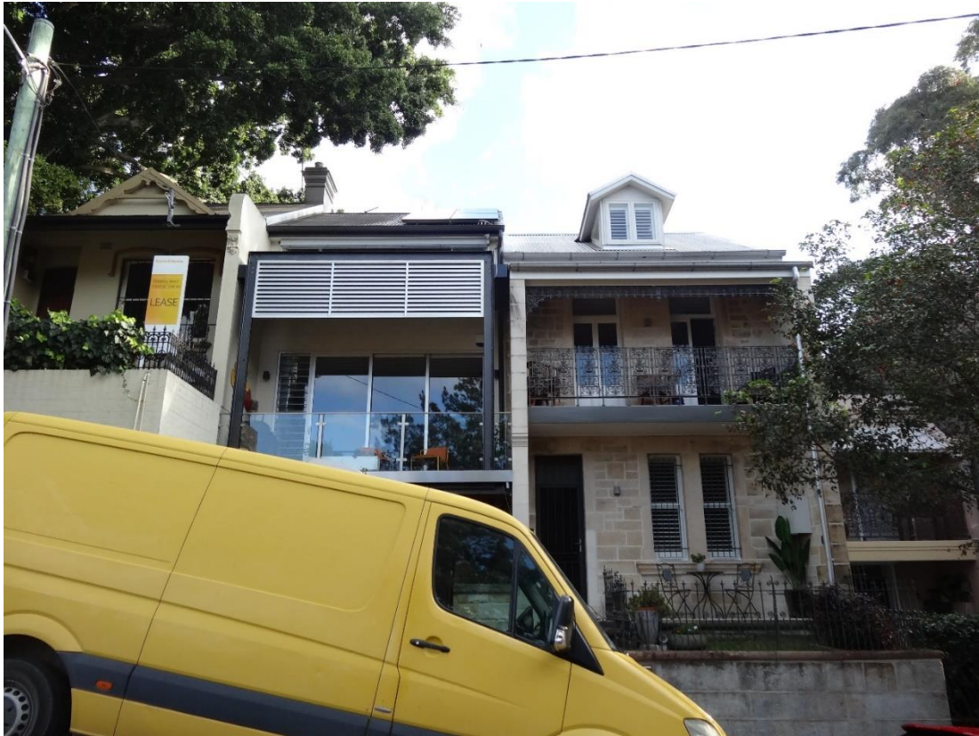
Figure 15: Residential terraces located on the opposite side of Bellevue Street
