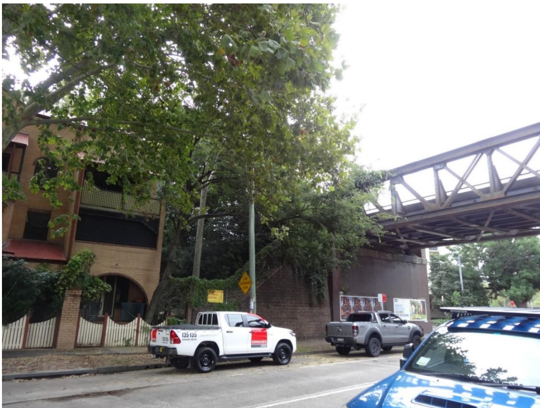
Figure 12: Light rail to the north of the site
